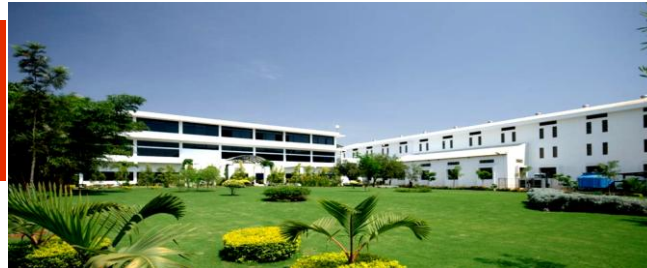
Unit I Factory
